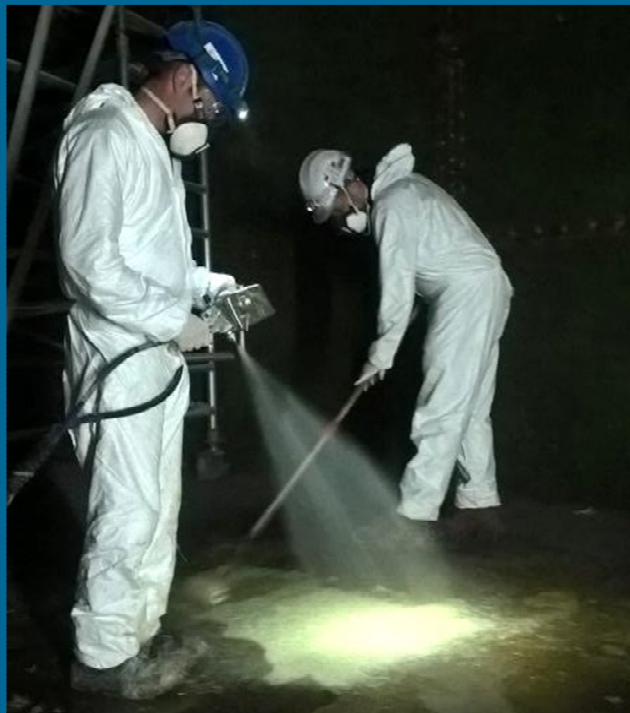
Formatank GRP liner applied using spray deposit technique to tank walls and base
