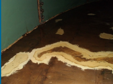
Concrete base existing damages
